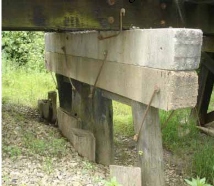
Typical Bent Section
