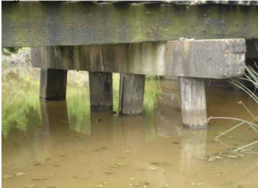
Typical Bent Section
