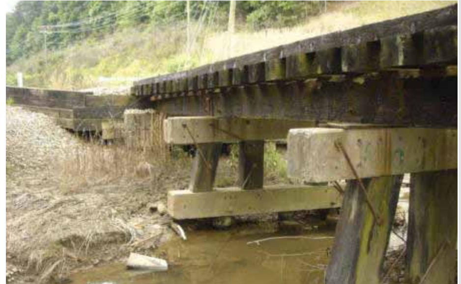
South Substructure View
