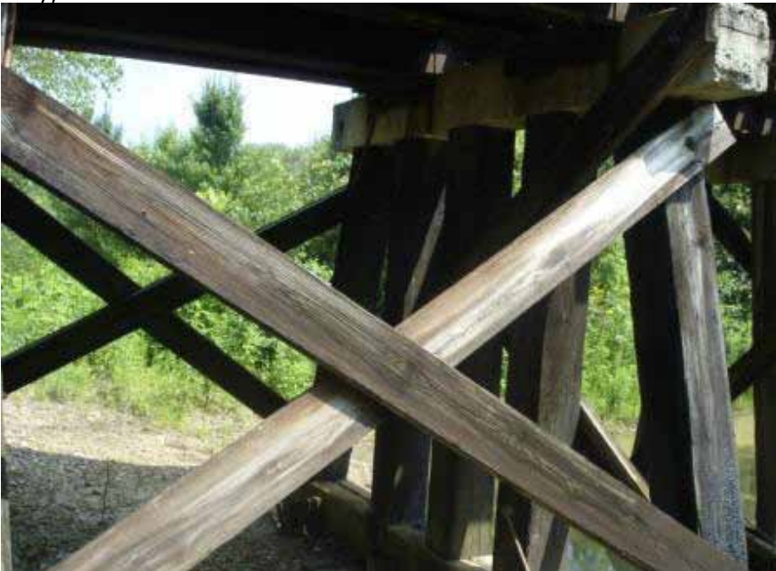
Typical Bent Cross Brace
