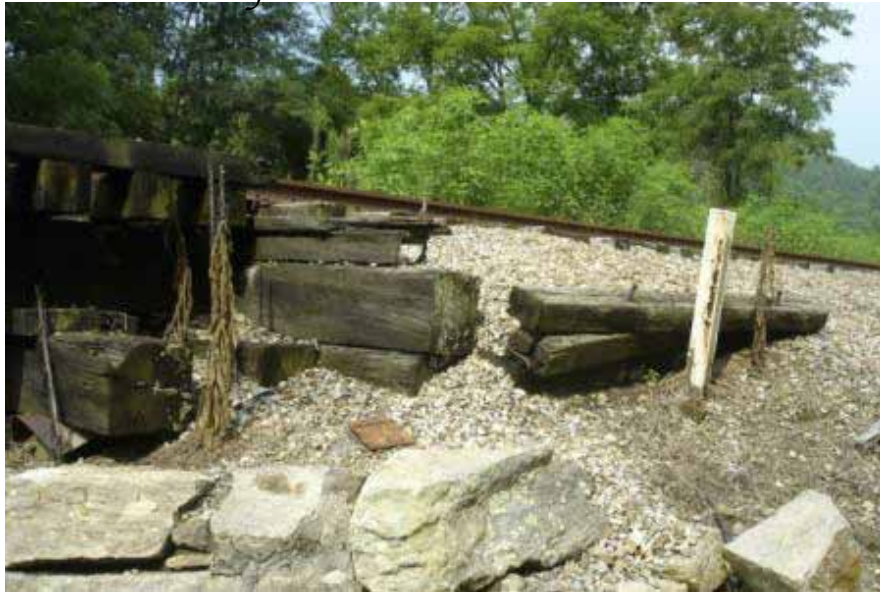
North Back Wall Undermining
