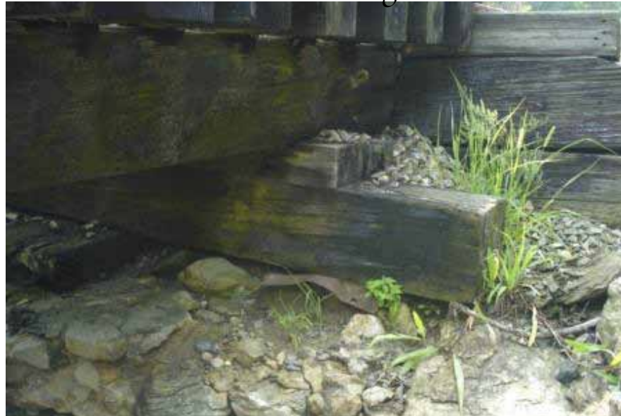
North Back Wall Undermining
