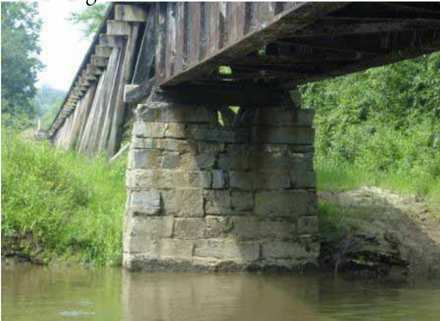
Steel Bridge Foundation
