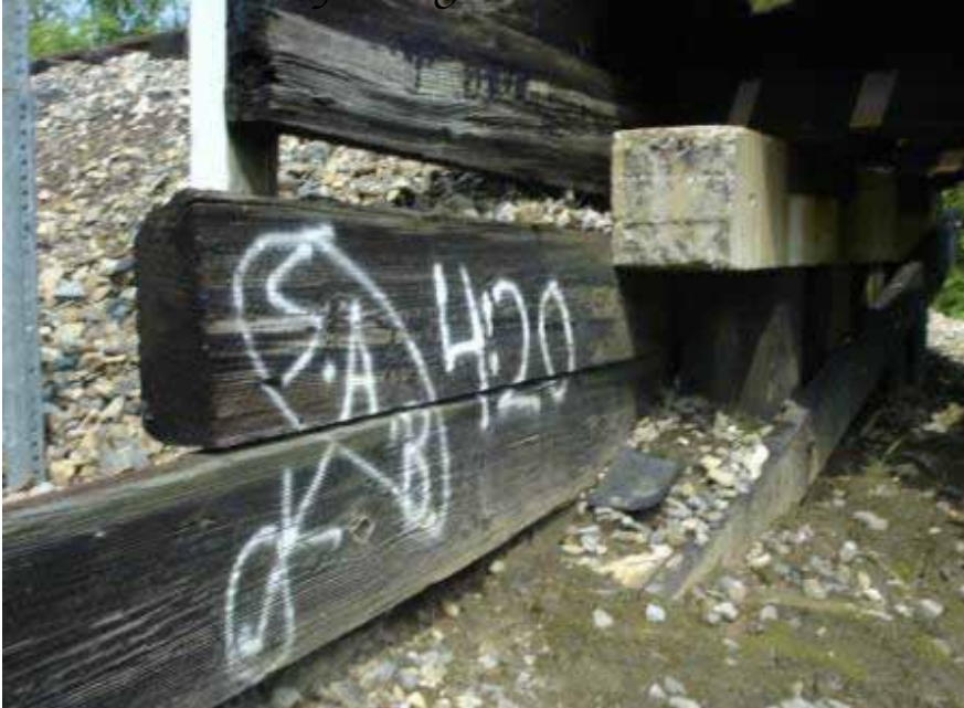
Typical Bent Cross Brace
