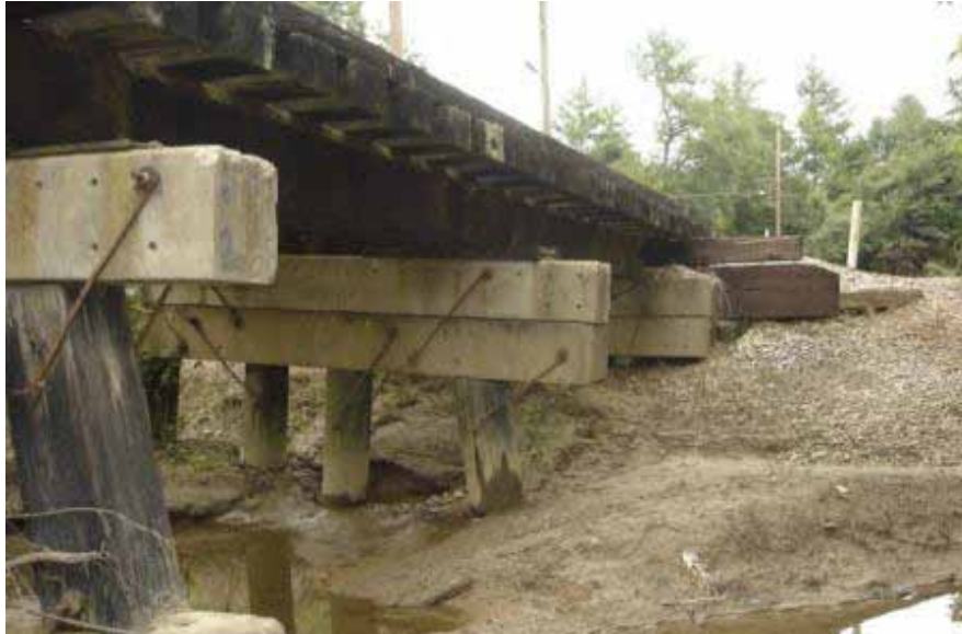
Typical Bent Section
