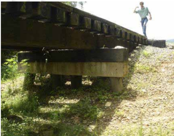
North Back Wall and Bent
