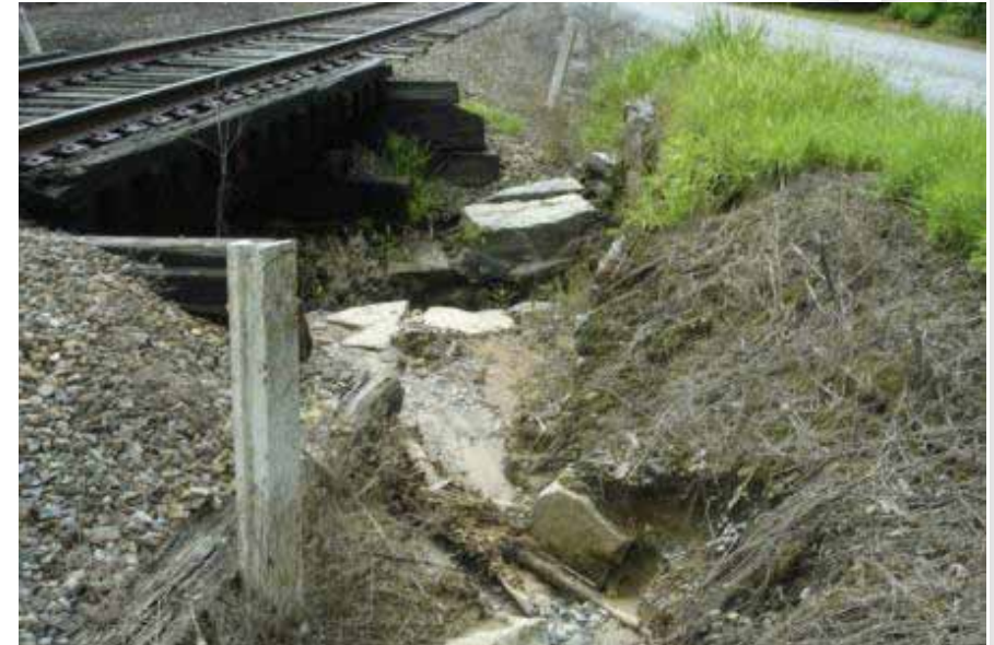
Severe Erosion
