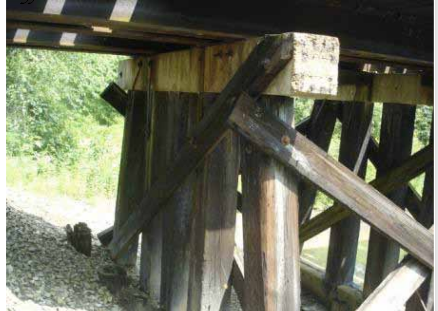
Bent Foundation Undermining
