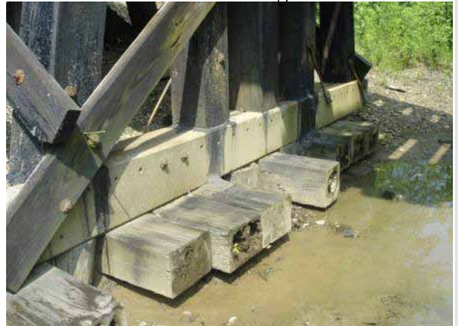
Bent Foundation Undermining
