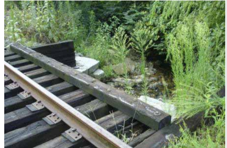
Tie and Timber Deterioration
